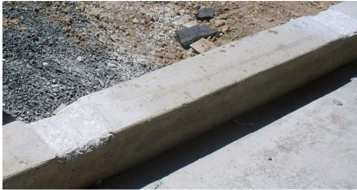
Figure 5.5: Chipped Concrete Curtain Wall Support Curb
