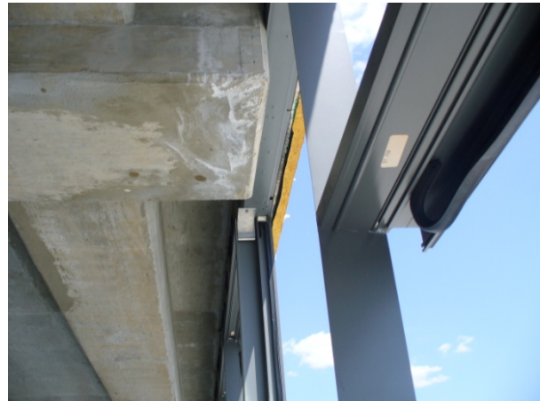
Figure 5.6: 7 th Floor PT Beams/Curtain Wall Conflict
